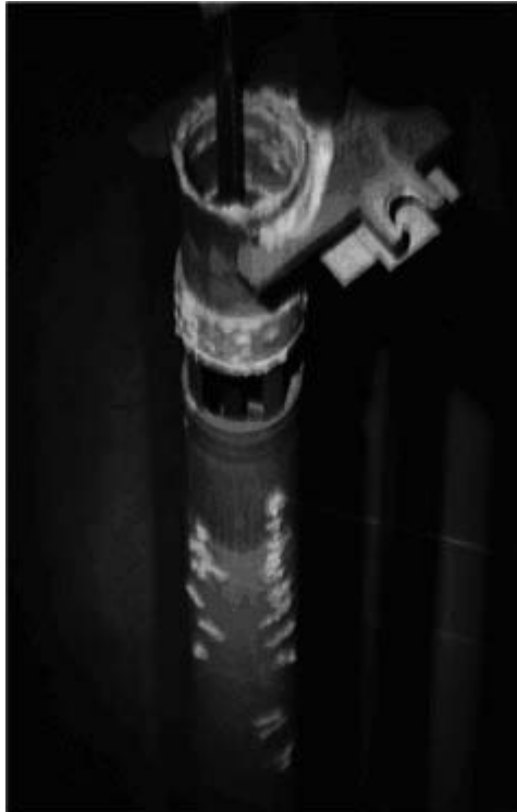
FIG 50. Mark-22 assembly in (aluminium) vertical tube storage with Type 304L stainless steel hangers. Aluminium corrosion products are at scratches on the outer surface of the Mark 22 and at the aluminium–stainless steel interface at the hanger.
