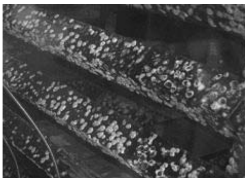
FIG. 52. SRS basin storage rack. Corrosion nodules from pitting corrosion of the aluminium storage racks after 35 years of basin service in water not optimized in chemistry control for aluminium corrosion.
